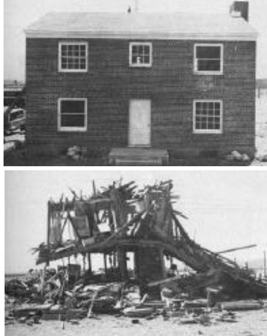
Above: Unreinforced brick house before a nuclear explosion at the Nevada Test Site. Below: Unreinforced brick house experiencing 5psi overpressure from a nuclear explosion at the Nevada Test Site. (Photo: US Federal Emergency Management Agency)
