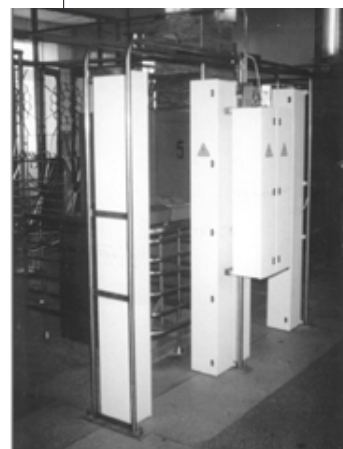
Pedestrian portal monitors at the Siberian Group of Chemical Enterprises Enrichment Plant. Photo.: Department of Energy
