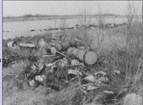
Contaminated rubble and soil from the demolition of a uranium processing facility and debris from a munitions factory and chemical plant have been dumped in Weldon Spring Raffinate Pit 4 in Missouri. Photo: US Department of Energy.
